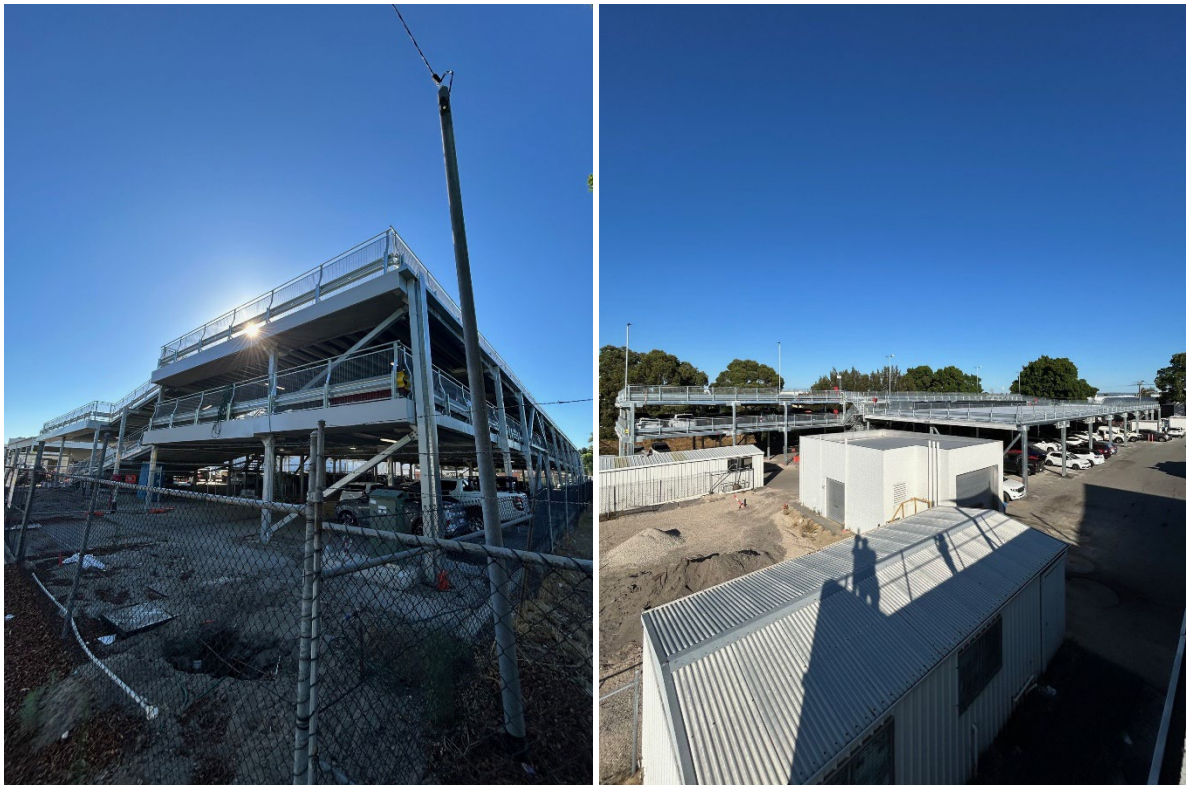
Figure 4 & 5: Substantial completion at Forward St
