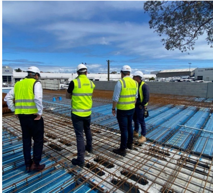
Figure 6: Inspection of installed works – Audi Myaree Project
