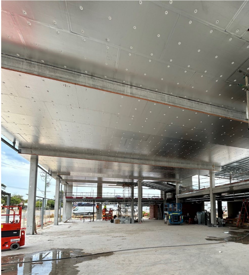
Photo 1. Image of CVB™xSimDek210™ spanning 18m at a height of 5.5m
