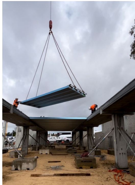
Above: Proof-of-Concept - MDSB® Application with SlimDek210®
