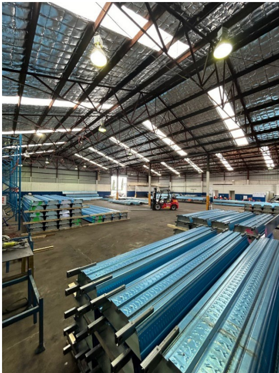
Above: Offsite Prefabrication MDSB® Assembly and Installation with SlimDek 210® | Fielders
