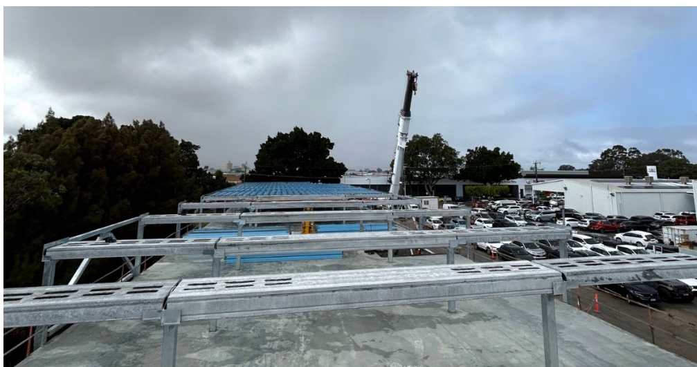
Figure 4: System Assembly at Forward St
