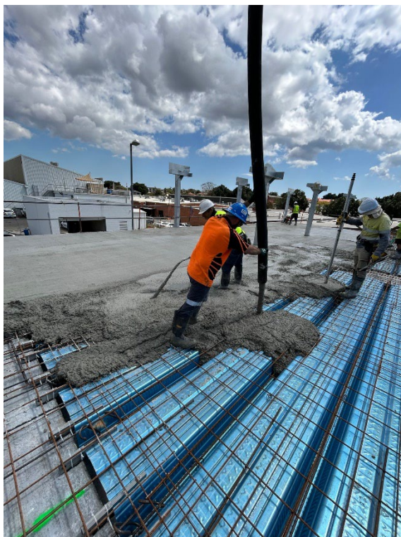
Figure 3: Suspended concrete works at Forward St
