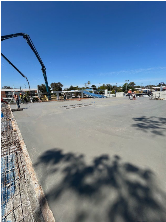
Figure 1: Suspended concrete works at Audi
