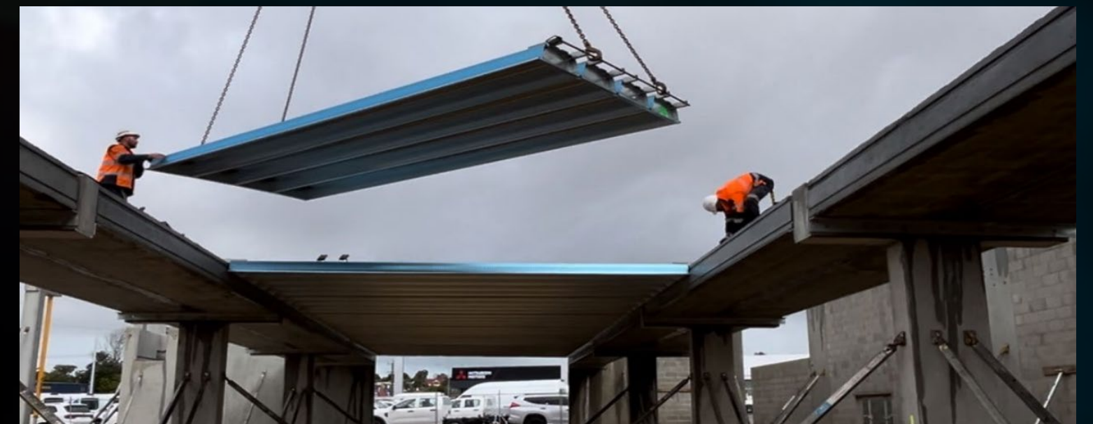
Installed CVB and Slimdek with MDSS in Perth, WA
