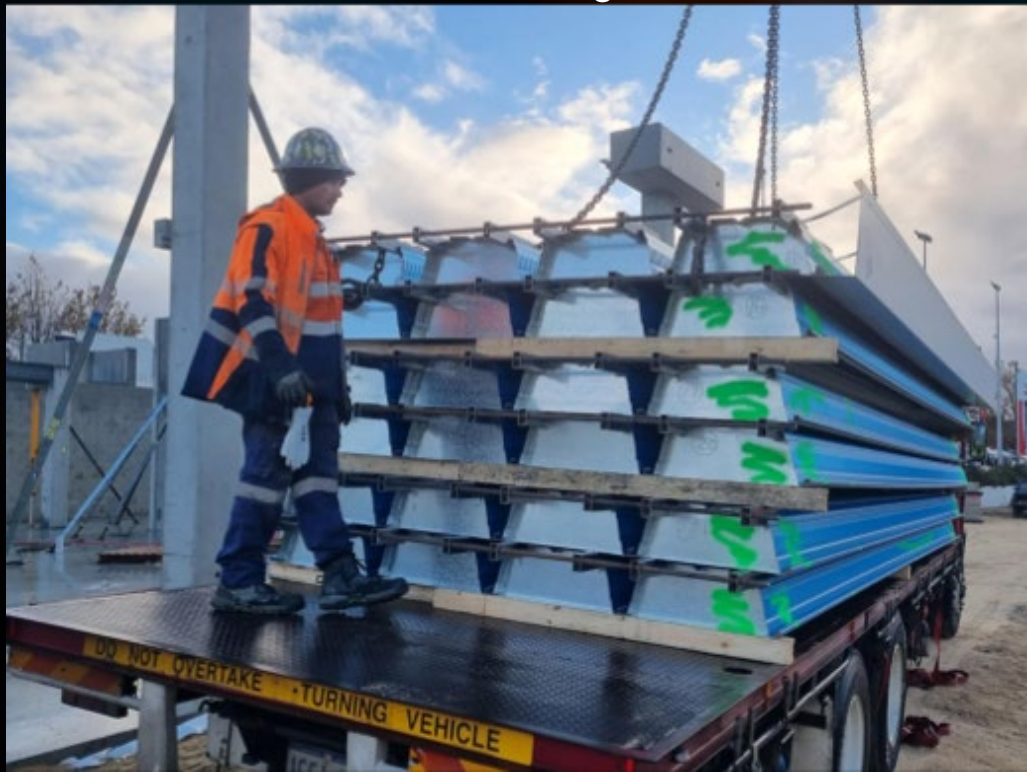
Slimdek prefabricated modules awaiting install
