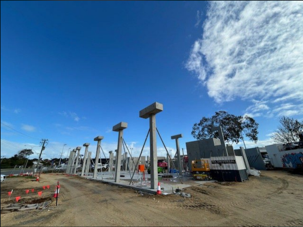
Columns installed at 6m in height
