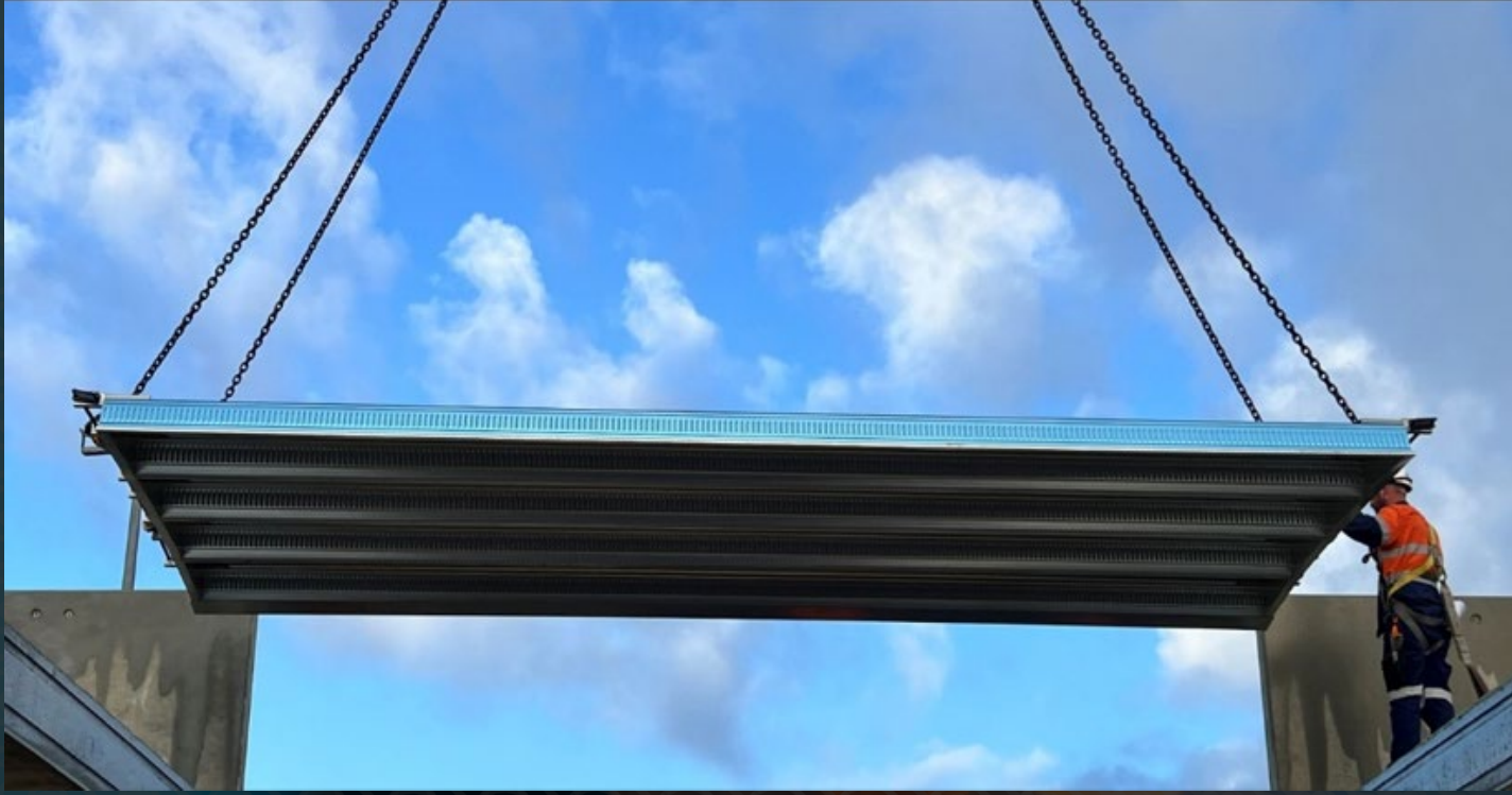
Slimdek module installation utilising the MDSB lifting bar
