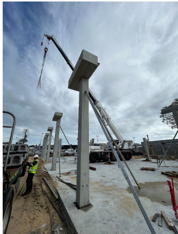
Figure 2: Construction at Audi Centre Myaree
