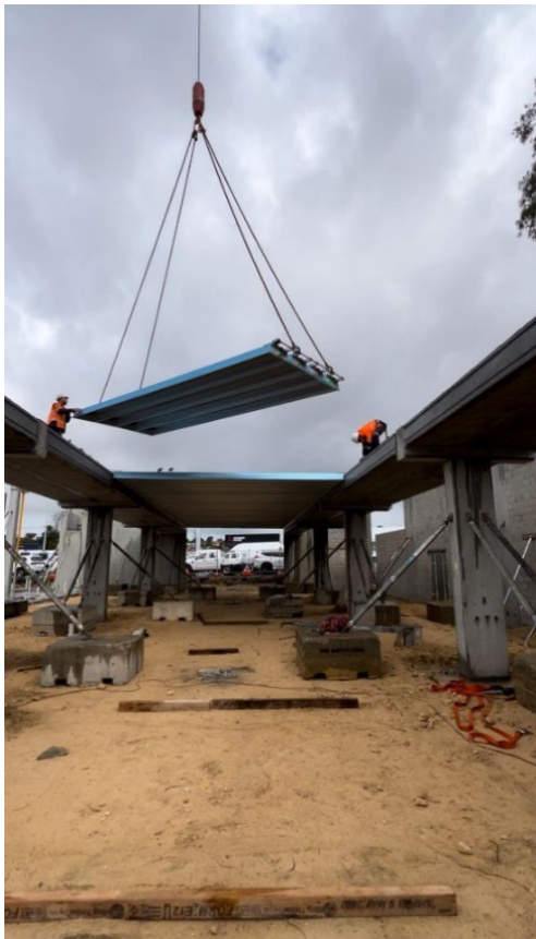
Figure 3 & 4. MDSS Installation at Audi Centre Myaree
